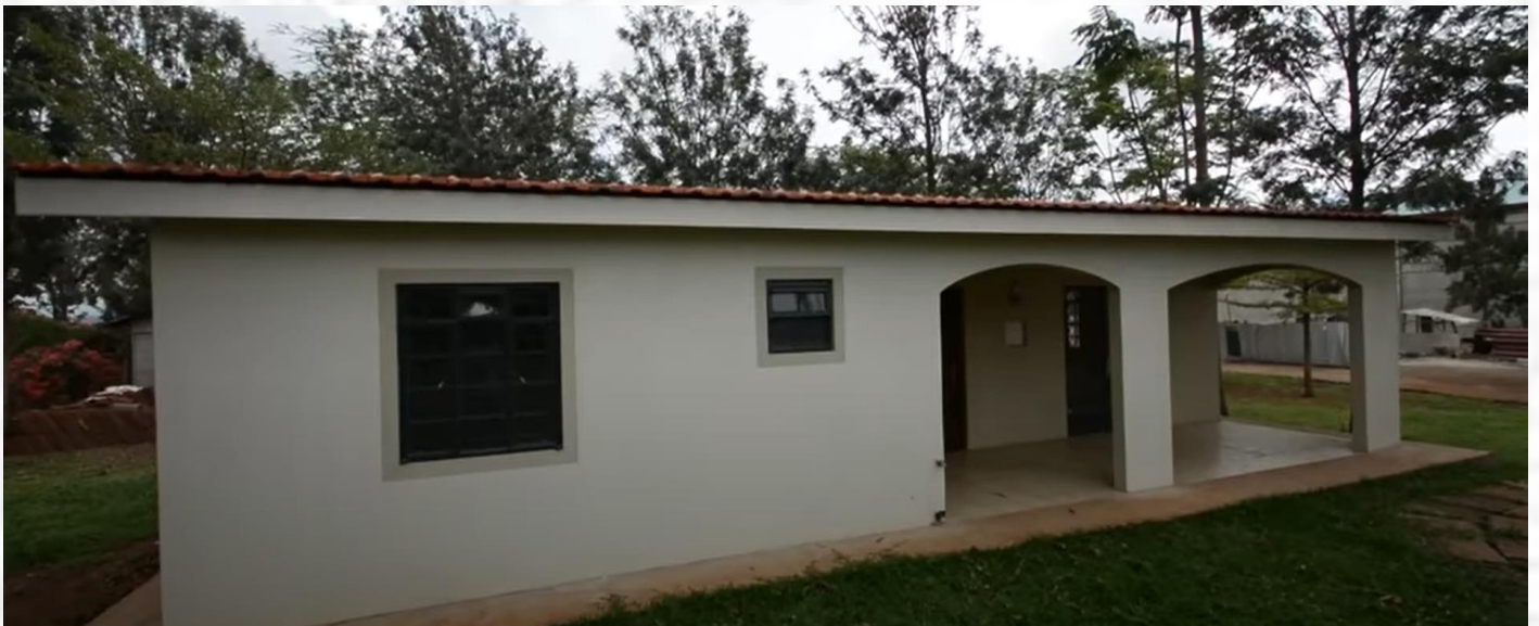
This residential development took 18 days
